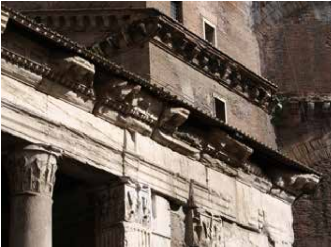
Plate 2 Pantheon, junction between the rotunda and transitional block at high level (Photo author)
