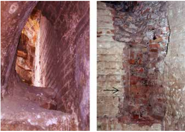
Plate 5 Pantheon, soundings made at the junction between the rotunda and the staircase wall running longitudinally on the side of the entrance in the transitional block. Left: east stair at high level; Right: west stair at low level (second landing). The arrow on the right-hand side image points to a course of two-foot wide bricks or bipedales , one of which traverses the junction whole and undamaged (photo: author)
