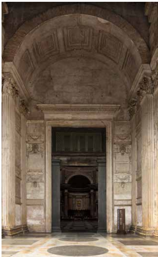
Plate 11a–b Pantheon, entrance and door. Note the pilasters and grille that fill the gap between the double doors and the masonry opening (a: photo: Maxim Atayants; b: Francesco Piranesi, Raccolta de' tempi antichi , II (1790), Tav. 20)
